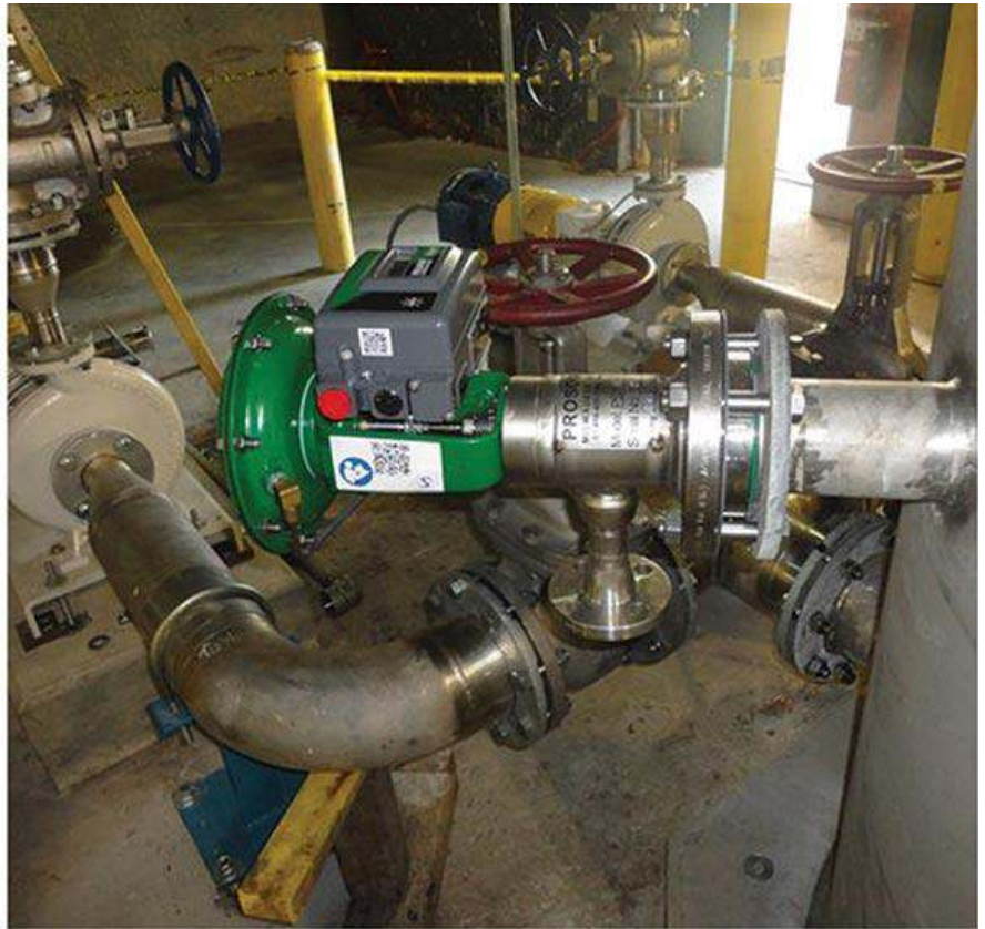
FIGURE 2. Different types of heaters have specific pressure-differential requirements. This is an example of radial multi-port jet diffuser design mounted on a hot water tank.
