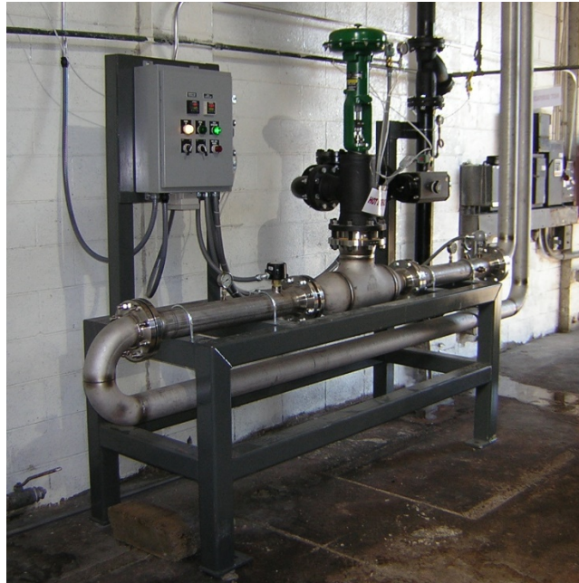
Figure 1: A very active hot water system where multiple users, such as hose stations, CIP spray nozzles and washdown areas, can put variable demand on the hot water system, which can impact the sizing of the system.
